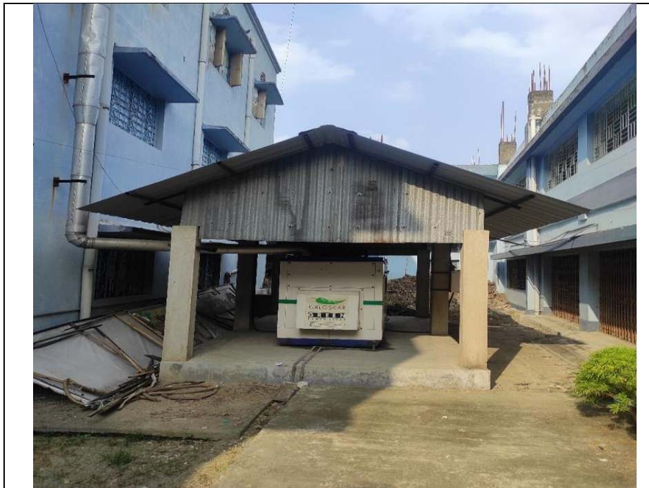
Silent DG sets are designed to generate a very low level of background noise, just as their name suggests. Their structures are constructed to eliminate virtually all noise and vibrations due to careful design. Because of this, they are not harmful to the environment and are ideally suited for use in residential areas.
