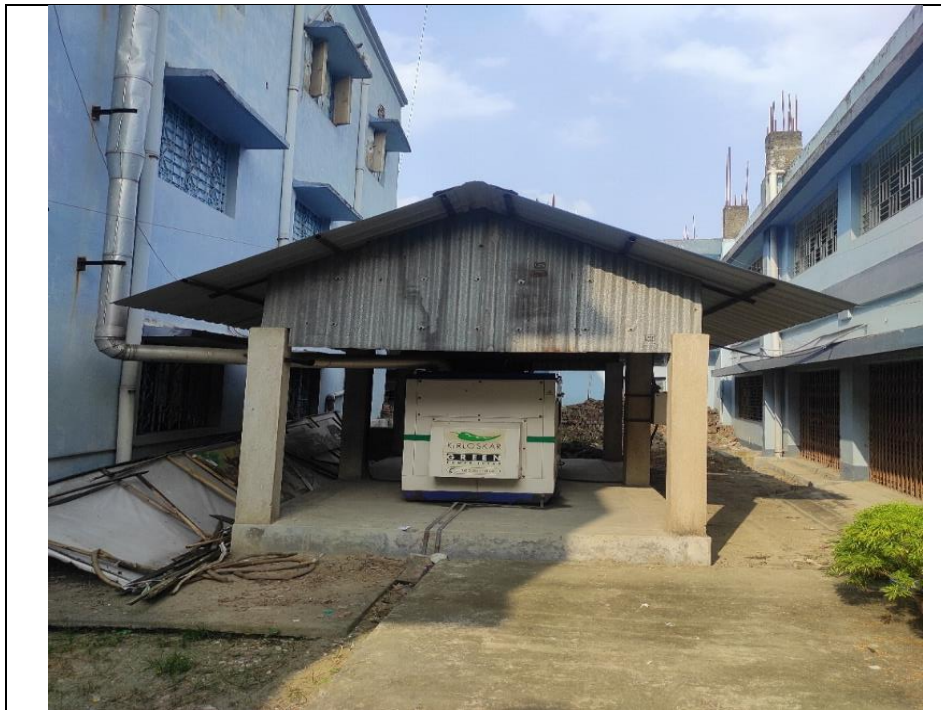
Silent DG sets are designed to generate a very low level of background noise, just as their name suggests. Their structures are constructed to eliminate virtually all noise and vibrations due to careful design. Because of this, they are not harmful to the environment and are ideally suited for use in residential areas.
